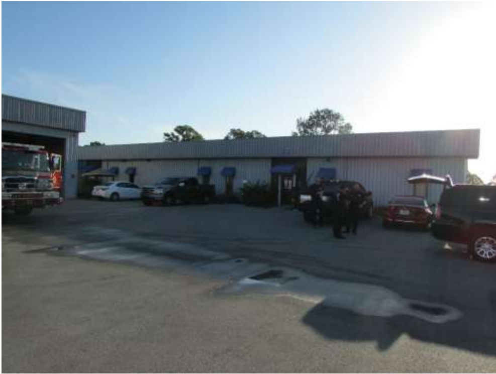
Front view of the administrative building (Photo Taken on April 6, 2021)
