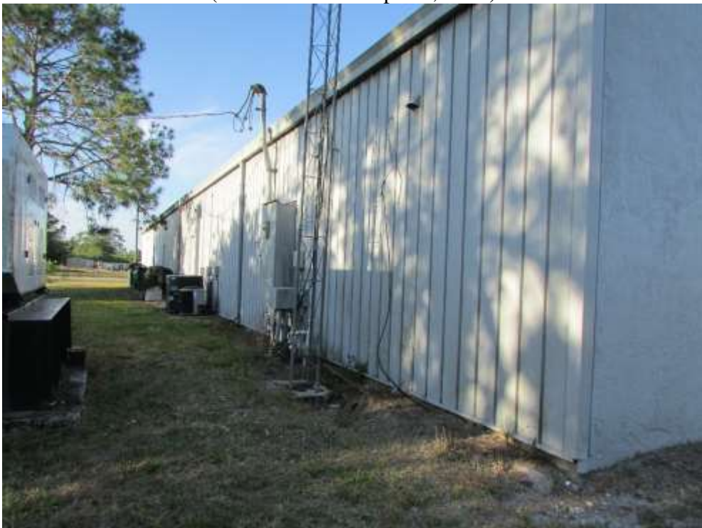
Rear view of the administrative building (Photo Taken on April 6, 2021)
