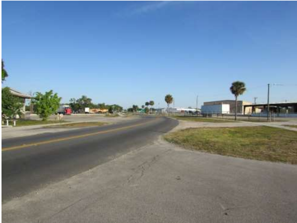
New Market Road looking northwesterly (Photo Taken on April 6, 2021)
