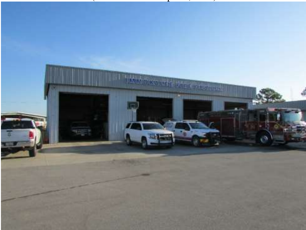
Front view of the apparatus bays (Photo Taken on April 6, 2021)
