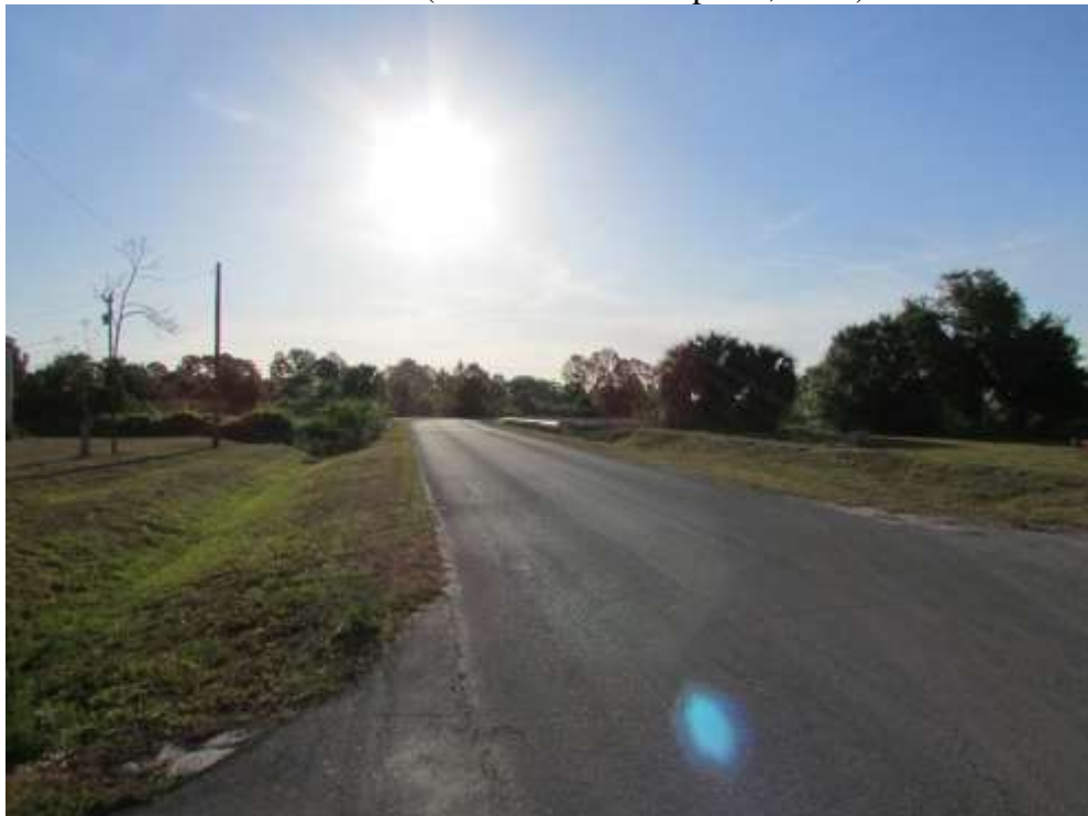
Airport Access Road looking easterly (Photo Taken on April 6, 2021)
